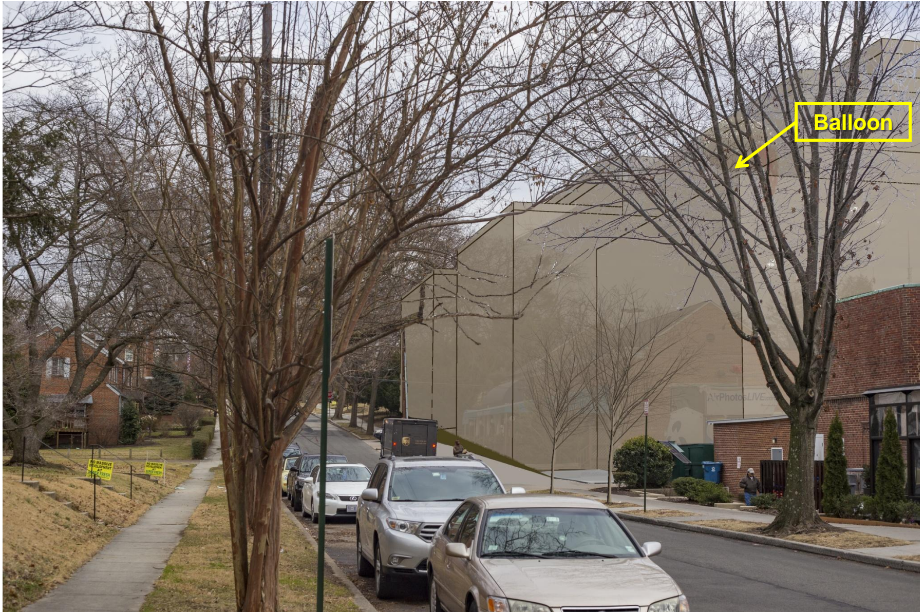
View from Camera Loc. 03. The 3D model-massing accurately represents the visual impact of the proposed development from this Yuma St perspective.
